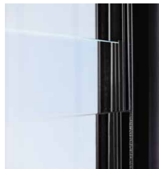
Traditional sashless window with single sheet of glass and overlapping panes when the window is in the closed position.
